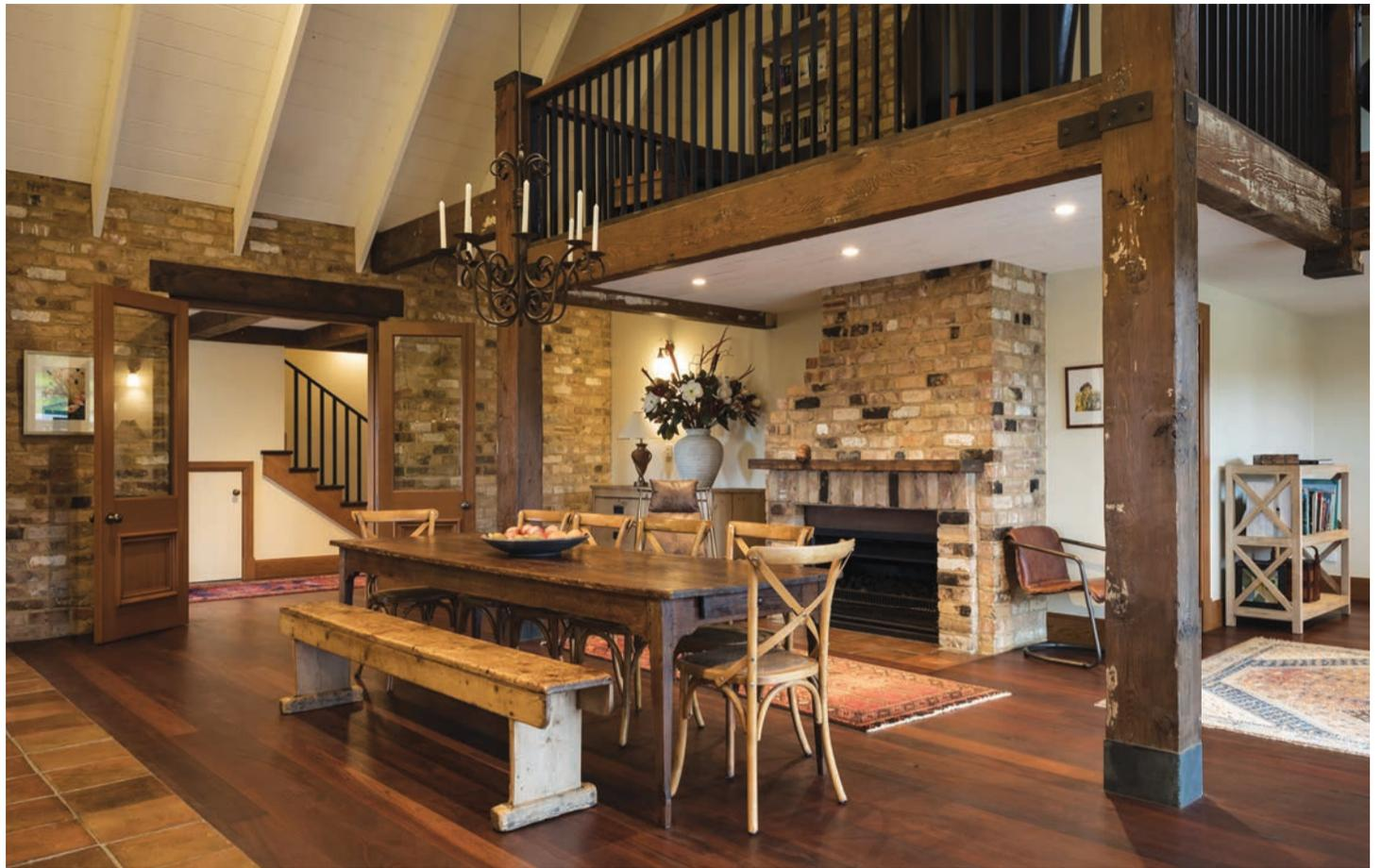
The interior is filled with recycled Oregon beams, exposed timber collar ties, macrocarpa sarking, French Oak architraves and skirting boards and Jarrah flooring throughout.
